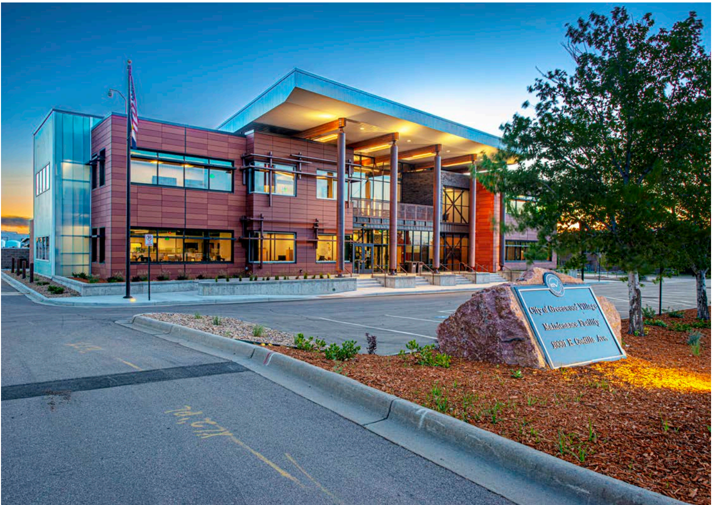
Greenwood Village Public Works Maintenance Administration Headquarters and Maintenance Facility.
